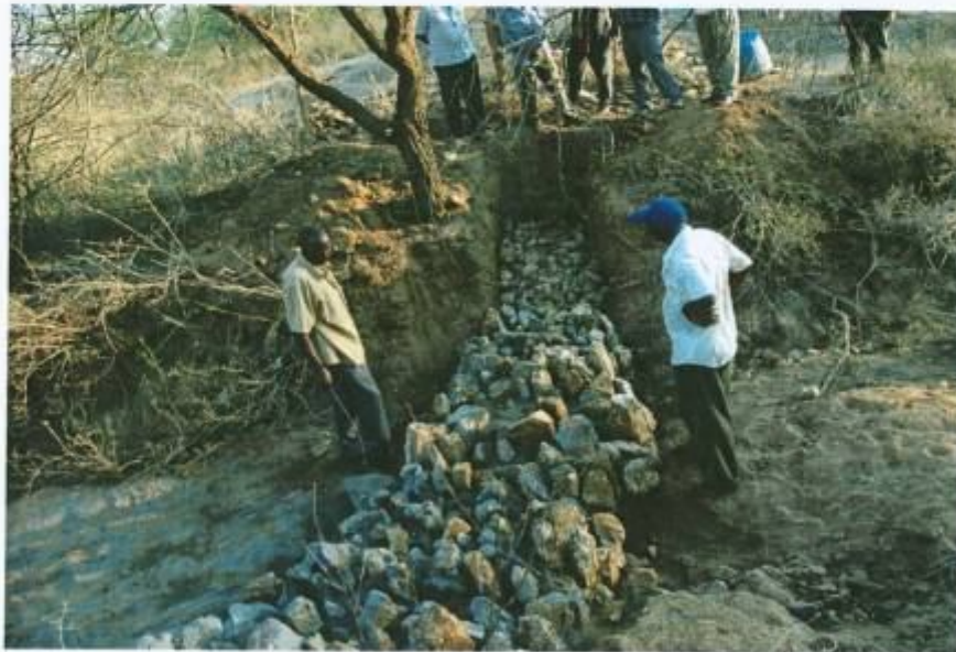
The photo below shows construction of check Dam. This is constructed to trap the silt and prevent sand from being washed into the reservoir .
